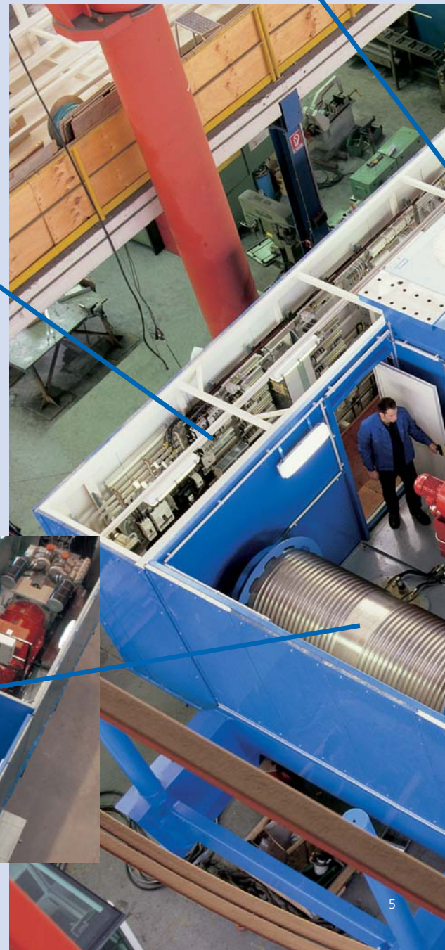
Superstructure with individual rooms, designed as modules
