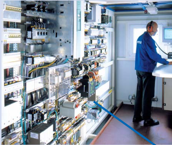
Air-conditioned electrics compartment
