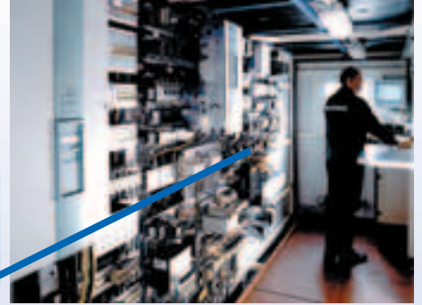
Air-conditioned electric compartment
