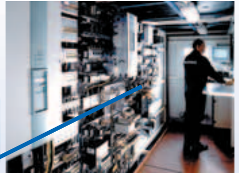
Air-conditioned electric compartment
